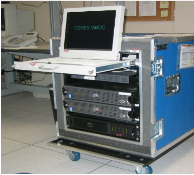
Figure 2 - Great Lakes Operations Center (VMOC at GRC)
